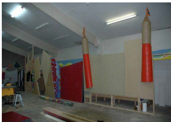
The Skate and Leisure Centre internal reconstruction project in progress.
